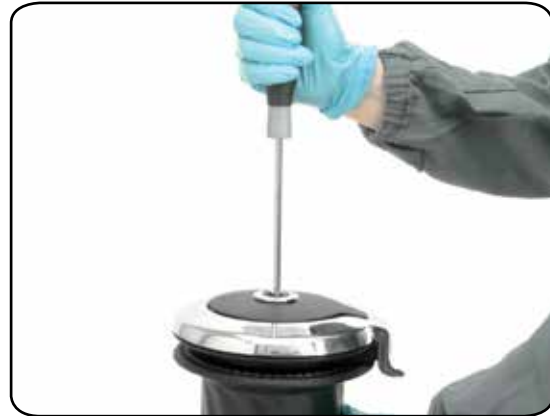
2. Unscrew the central screw ( \approx 2\text{Nm}/18\text{ in-lb} )
