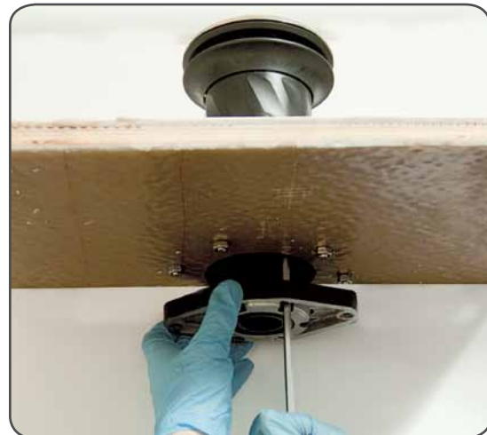
2. Tighten the six screws ( \approx 8 Nm/ 71 in-lb)
